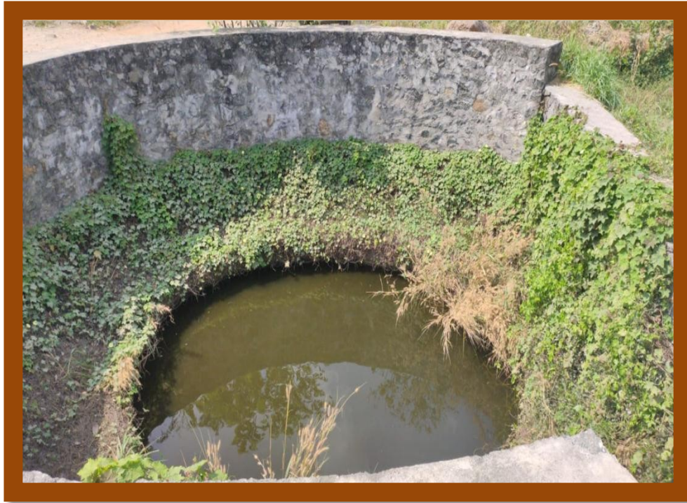
RAINWATER HARVESTING PIT
